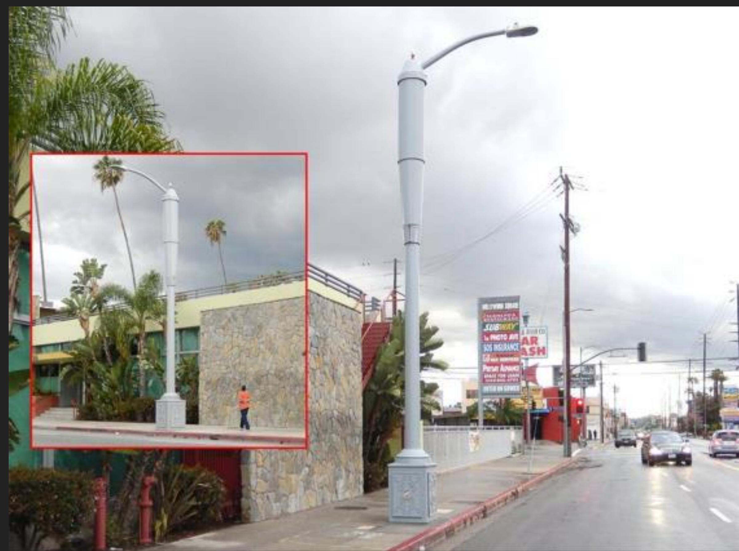
Phillips/Ericsson "ZeroSite" | Composite Pole with panel antennas inside and equipment in base | Considered too large for most small-scale streets
